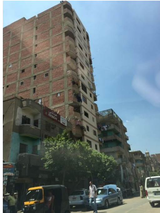
Figure 31 Another tower with unfinished side walls (Author, 2015)
