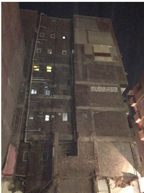
Figure 52 Building with obvious tilt in the last three floors (Author, 2015)
